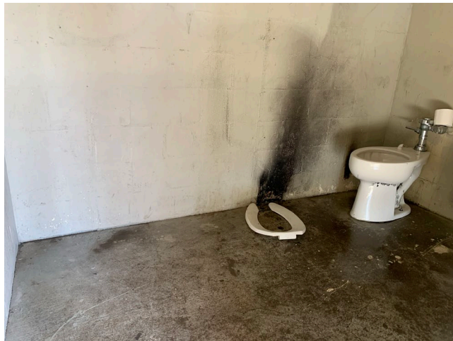
Photo 15 – Restroom building #2 interior
