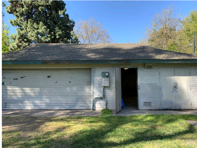
Photo 19 – Maintenance building, non-asbestos-containing CMU mortar, concrete and roofing materials
