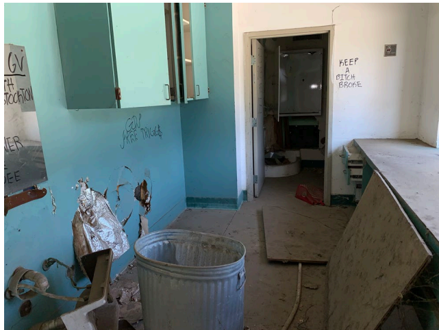
Photo 3 – Bath house interior non-asbestos-containing gypsum wallboard system, baseboard mastic and concrete
