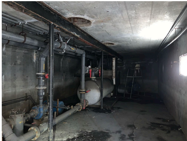
Photo 6 – Basement pool pump room, non-asbestos-containing concrete
