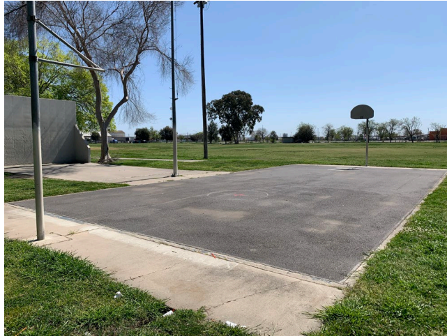
Photo 10 – Basketball and handball courts, non-asbestos-containing concrete and asphalt
