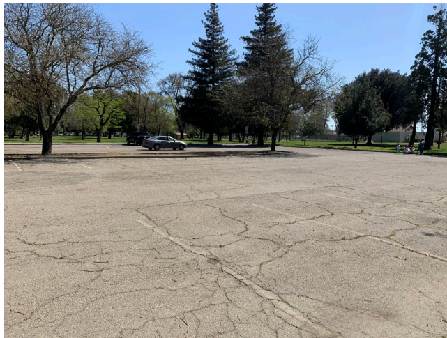
Photo 8 – Parking lot, non-asbestos-containing asphalt
