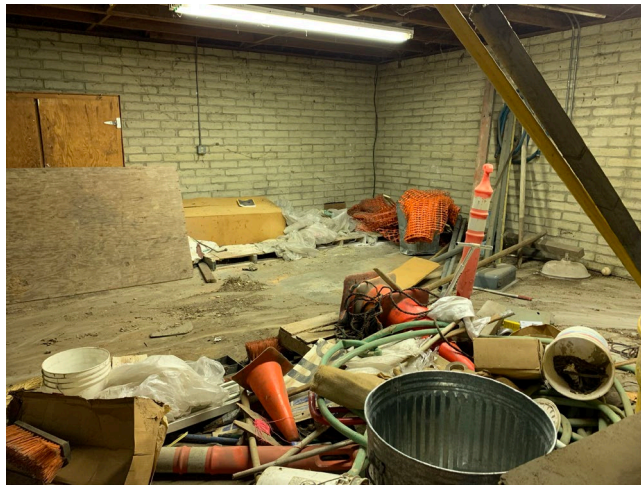
Photo 20 – Maintenance building, interior
