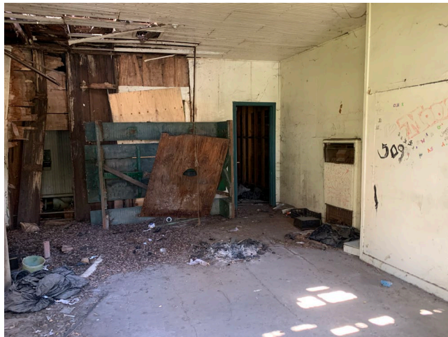
Photo 18 – Park personnel building, interior
