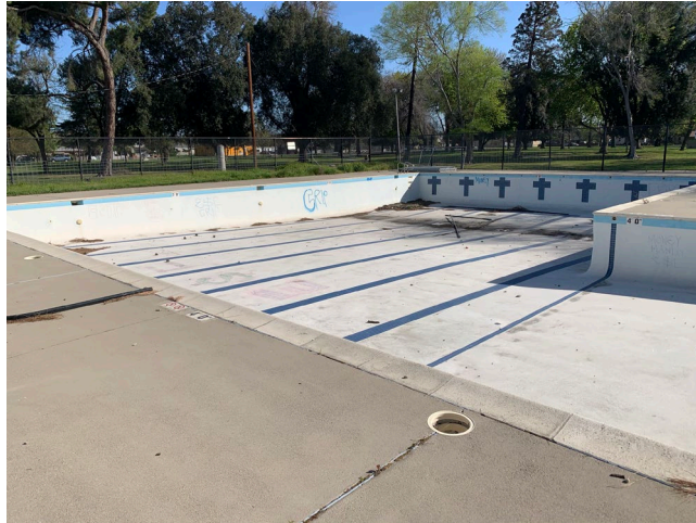
Photo 4 – Swimming pool, non-asbestos-containing concrete and pool coating
