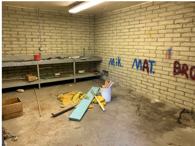
Photo 21 – Maintenance building, interior
