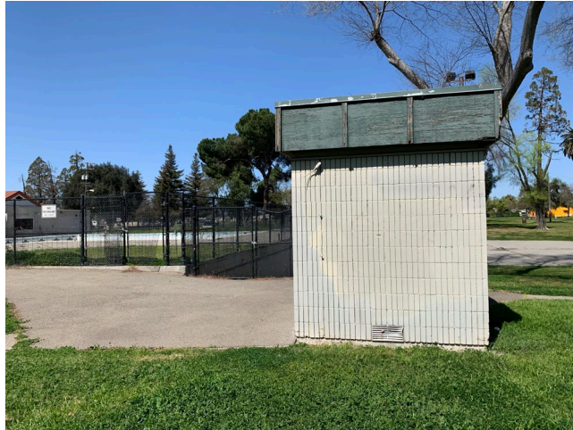
Photo 7 – Pool chemical storage building
