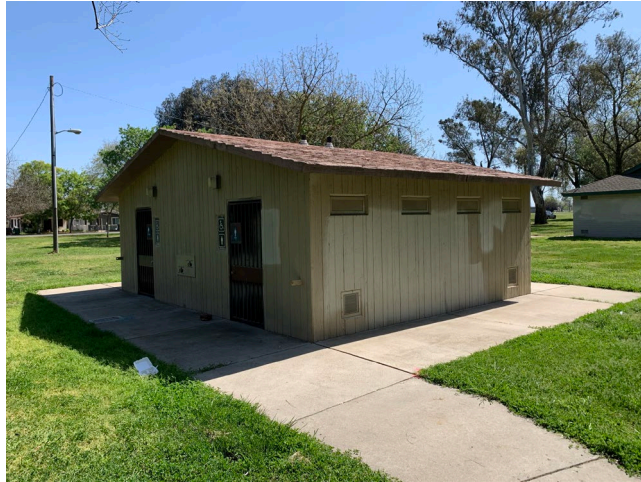
Photo 13 – Restroom building #1, non-asbestos-containing concrete floor, walls and roof
