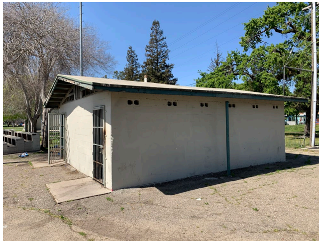
Photo 14 – Restroom building #2, non-asbestos-containing concrete, CMU mortar and roofing materials
